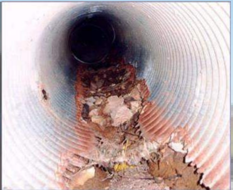
Complete failure due to corrosion
