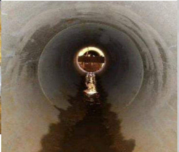
Complete failure due to corrosion
